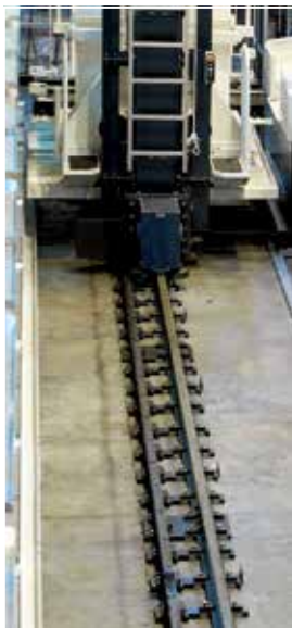
Cableless Data Communications
